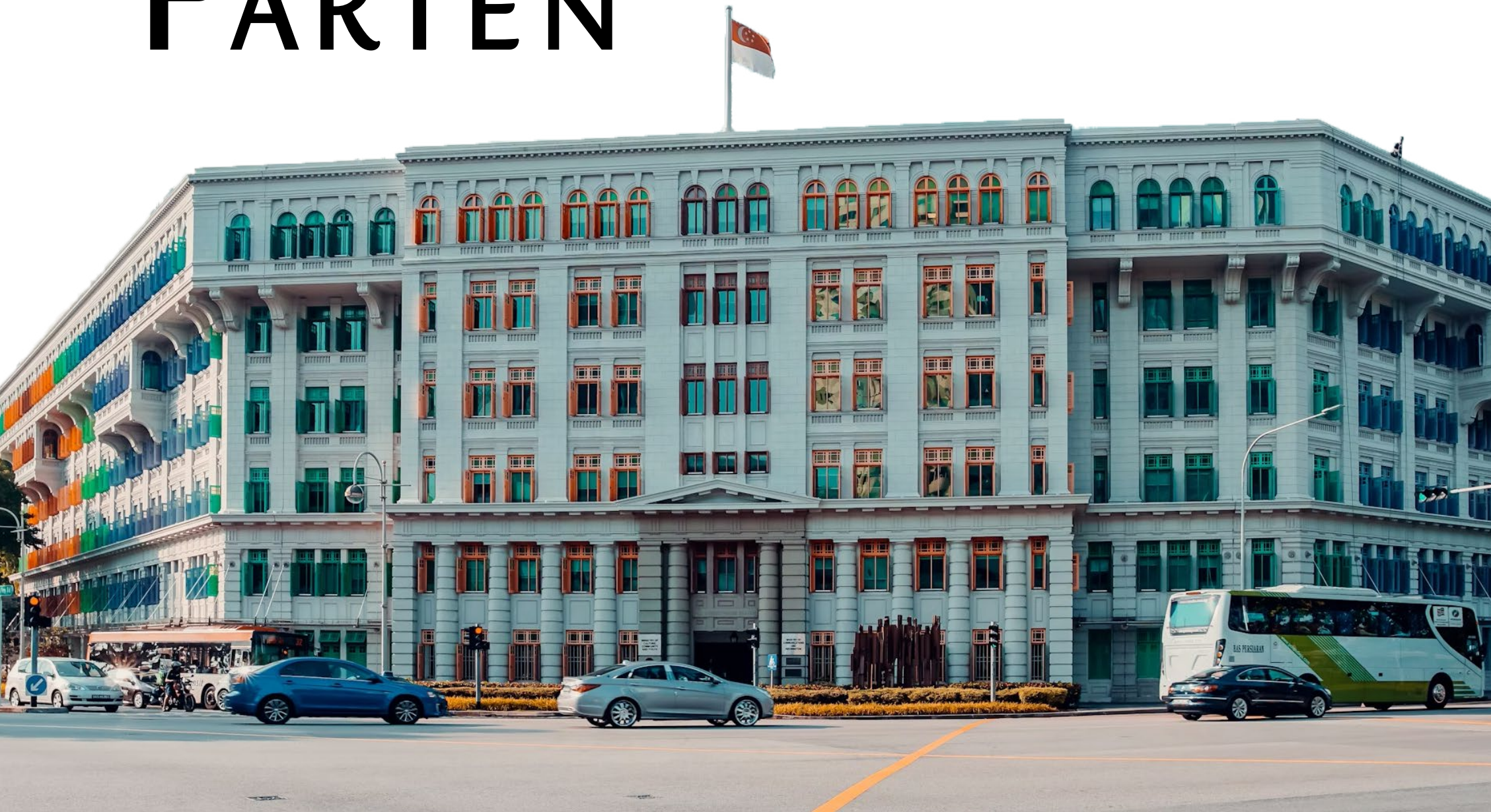
Old Hill Street Police Station, Singapur
